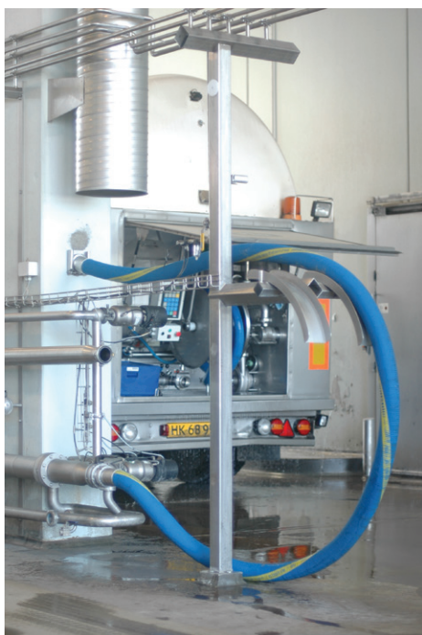
Raw material intake
